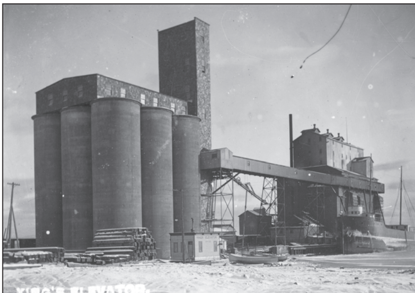
King's Hospital Elevator, 1906. These nine cylindrical reinforced concrete bins built in 1903 using Haglin's slip-form method of concrete construction are the first known concrete silos to have been erected in Canada for a grain elevator. The 1883 wood crib elevator (at right) was demolished in May 1923. (Vervoort, 1990, below). TBHMS 975.1.597.
