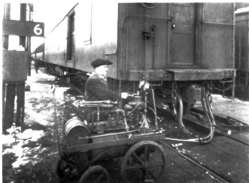
Glen Yard employee testing brakes on passenger cars. From Canadian Pacific Corporate Archives, photo 12800.
