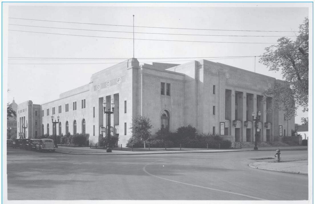
FIG. 14. WINNIPEG AUDITORIUM, NORTHWOOD AND CHIVERS, SEMENS, PRATT AND ROSS, BUILT 1932. CITY OF WINNIPEG ARCHIVES. CITY OF WINNIPEG ARCHIVES PHOTOGRAPH COLLECTION (P02 FILE 26), [HTTPS:// WINNIPEGINFOCUS.WINNIPEG.CA/I01428].
