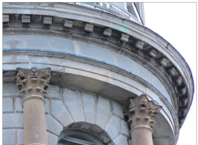
FIG. 49. ST. GEORGE'S CHURCH, BELFRY, 1842; DETAIL OF CORINTHIAN CAPITALS AND ENTABLATURE. | PHOTO: PAUL CHRISTIANSON, JULY 2022.
