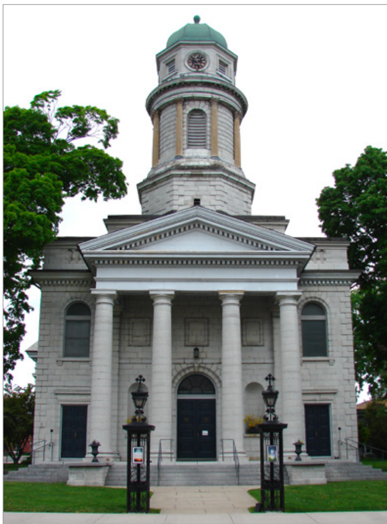
FIG. 32. ST. GEORGE'S ANGLICAN CHURCH, RITUAL WEST FAÇADE WITH PORTICO AND TOWER 1842-1847. | PHOTO: PAUL CHRISTIANSON, MAY 2020.
