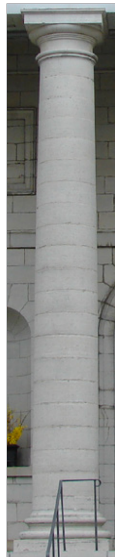
FIG. 34. ST. GEORGE'S CHURCH; DETAIL OF MODIFIED TUSCAN COLUMN, 1842. | PHOTO: PAUL CHRISTIANSON, JANUARY 2021.
