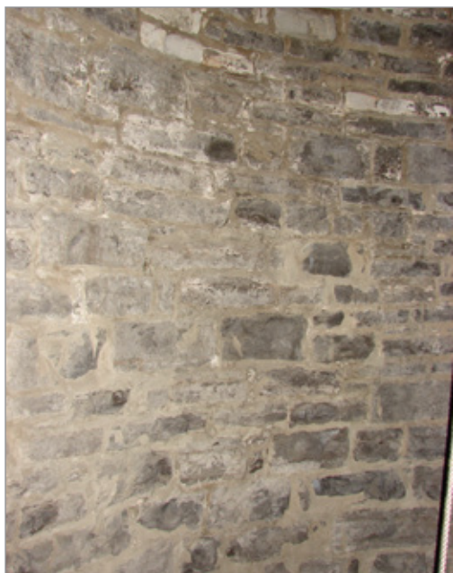
FIG. 17. ST. GEORGE'S CHURCH, 1839-1841; DETAIL OF INTERIOR OF TAPERED CIRCULAR WALL FROM TOP OF NARTHEX TO FLOOR OF THE BELFRY. | PHOTO: PAUL CHRISTIANSON, NOVEMBER 2020.
