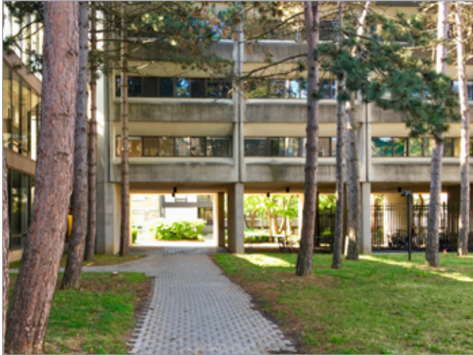
FIG. 19. NORTHERN COURTYARD OF MACKINTOSH-CORRY HALL (R.J. THOM ARCHITECTS, 1972-1974), QUEEN'S UNIVERSITY, KINGSTON. | JAMES ASHBY, 2019.
