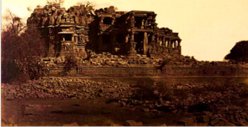
FIG. 3. THE TWELFTH-CENTURY NAVALAKHA TEMPLE, GHUMLI, GUJARAT, INDIA, SEEN FROM THE SOUTH IN 1874. | JAMES BURGESS AND JOHN FAITHFULL FLEET, 1971 [1876], REPORT ON THE ANTIQUITIES OF KATHIAWAD AND KACHH, BEING THE RESULT OF THE SECOND SEASON'S OPERATIONS OF THE ARCHAEOLOGICAL SURVEY OF WESTERN INDIA, 1874-75 , VARANASI, INDOLOGICAL BOOK HOUSE, PLATE XL.
