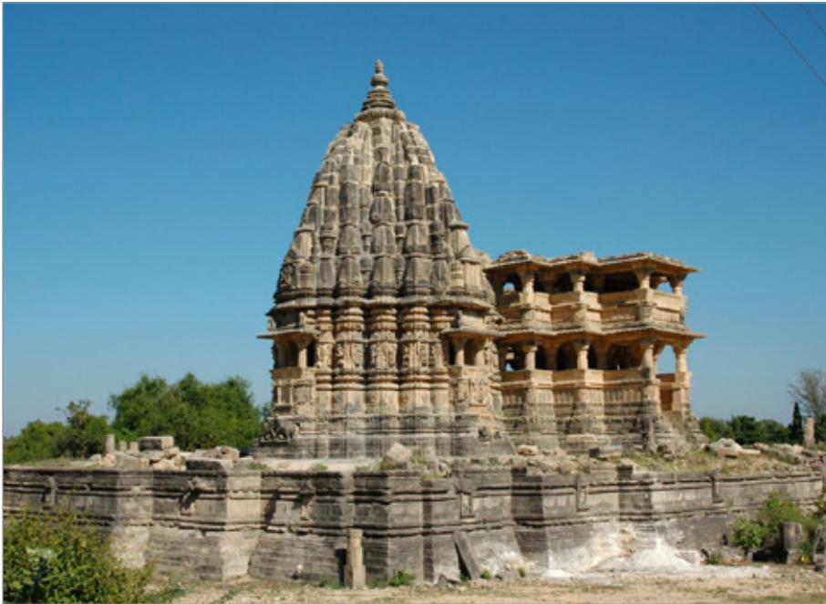
FIG. 4. PHOTOGRAPHED FROM THE SOUTH-WEST, THE NAVALAKHA TEMPLE, GHUMLI, GUJARAT. RESTORED BY THE ARCHAEOLOGICAL SURVEY OF INDIA IN 2011, THE TEMPLE PROPER IS ON THE LEFT, AND A TWO-STOORY MAṄḌAPA IS ON THE RIGHT. | LIBBIE MILLS, DECEMBER 2010.
