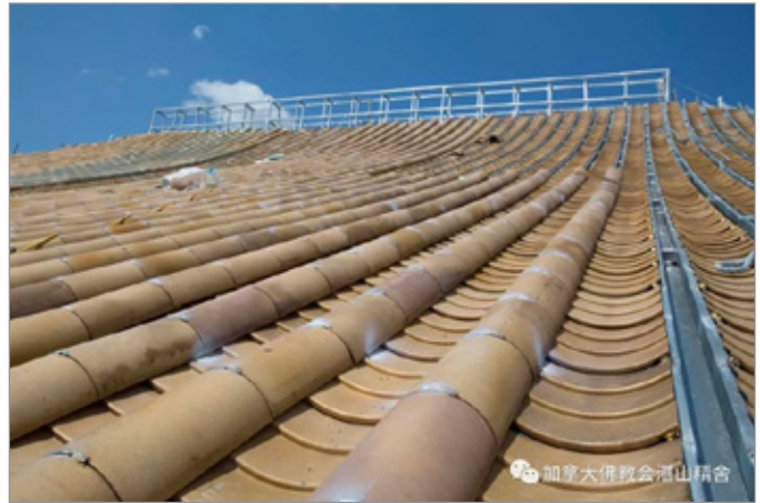
FIG. 23. COPPER TILES COVER THE ROOF THE MAIN DARMA HALL AT THE WUTAI SHAN BUDDHIST GARDEN, 708 SKI HILL ROAD, BETHANY, ON. | BUDDHIST ASSOCIATION OF CANADA'S CHAM SHAN TEMPLE: [HTTP://THEBUDDHISTGARDEN.COM/GALLERY%E7%9B%B8%E7%89%87%E9%9B%86/COPPER-TILED-ROOF-%E5%A4%A7%E6%AE%BF%E9%8A%85%E7%93%A6%E5%BB%BA%E8%A8%AD%E5%B7%A5%E7%A8%BB/], ACCESSED AUGUST 24, 2021.
