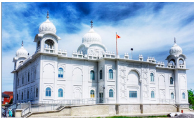
FIG. 37. THE DASHMESH DARBAR, 555 EBENEZER ROAD, BRAMPTON, ON: [HTTPS://WWW.FLICKR.COM/PHOTOS/15546179@N08/14160104469]. | PAUL VAN DAMME, JUNE 2014.
