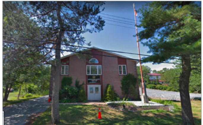
FIG. 30. THE GURDWARA OF THE MARITIME SIKH SOCIETY (1978), 10 PARKHILL ROAD, HALIFAX, NS: [HTTPS://WWW.GOOGLE.CA/MAPS/@44.6243341,-63.6006573,3A,75Y,309H,100.82T/DATA=!3M6!1E!13M4!1STMLUGSIZTGCK7RNKYFW4HQ!2E0!7!16384!8!8192?HL=EN]. | GOOGLE MAPS.
