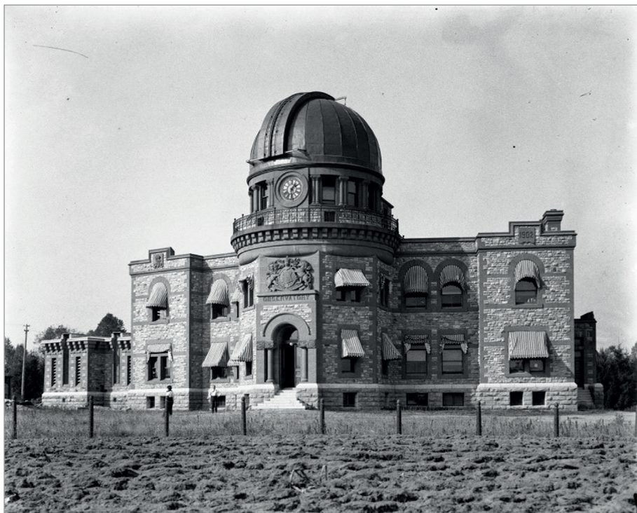
FIG. 5. DOMINION OBSERVATORY, OTTAWA CONSTRUCTION, FRONTAL VIEW, C. 1904. | SLIDE 311-3, DOMINION OBSERVATORY COLLECTION, NATURAL RESOURCES CANADA ARCHIVES, EARTH SCIENCES DEPARTMENT.
