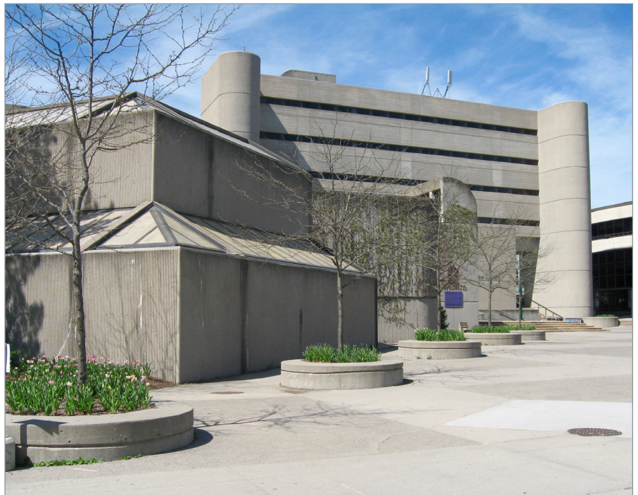
FIG. 9. THE SANDBLASTED, STRIATED CONCRETE WALLS OF THE D.B. WELDON LIBRARY (MURPHY, SCHULLER, GREEN, & MARTIN, AND JOHN ANDREWS ARCHITECTS), 2013, WESTERN UNIVERSITY, LONDON. | PHOTO: JAMES ASHBY.
