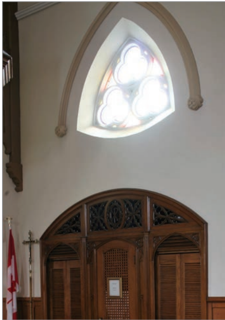
FIG. 55. NIAGARA FALLS, ST. PATRICK, INTERIOR, PENULTIMATE N (S) BAY. | MALCOLM THURLBY.
