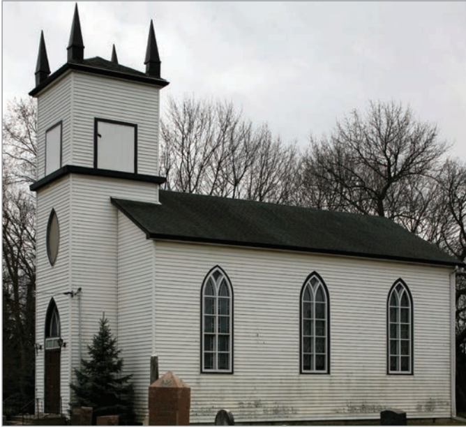
FIG. 13. PORT ROBINSON, ST. PAUL'S ANGLICAN CHURCH (1844), EXTERIOR FROM SW. | MALCOLM THURLBY.
