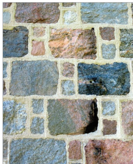
FIG. 17. CRELLIN'S ABERDEEN BOND STYLE MASONRY WITH 2 SNECKS, MCCOMB HOUSE, I 33 RD LINE, NO. 6603, NEAR HARRINGTON, OXFORD COUNTY. | KAREN E. ARMSTRONG.
