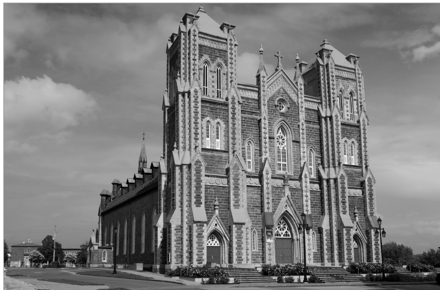
FIG. 19. CHURCH OF LA NATIVITÉ DE NOTRE-DAME, BEAUPORT (BUILT 1916-1918), EXTERIOR VIEW. TANGUAY ET LEBON, ARCHITECTS. | MARC GRIGNON, 2017.
