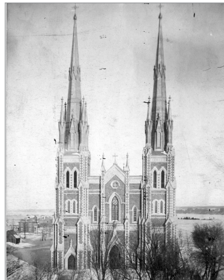
FIG. 14. VIEW OF THE FOURTH CHURCH OF LA NATIVITÉ DE NOTRE-DAME, BEAUPORT (PHOTO C. 1916). FRANÇOIS-XAVIER BERLINGUET, ARCHITECT (BUILT 1890-1892, DESTROYED 1916). | UNKNOWN PHOTOGRAPHER. BANQ, COLLECTION CENTRE D'ARCHIVES DE QUÉBEC, FONDS RAOUIL CHÉNEVERT, P372,D44,P1.
