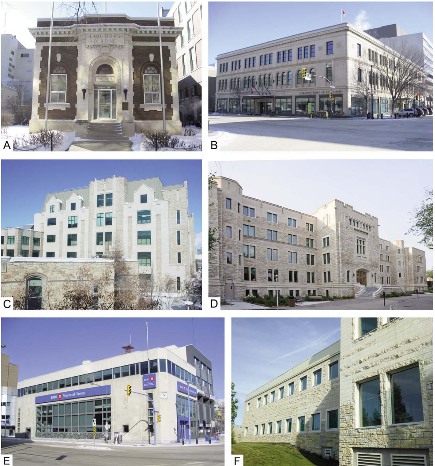
Figure 29. Examples of the range of building styles using Tyndall Stone, Saskatoon. A. Land Titles Building (1910). Neo-classical and neo-Romanesque. B. Eaton's Building (1928). Neo-Renaissance style. C. Spinks Addition to Chemistry Building, University of Saskatchewan (2003). Châteauesque style. D. Health Sciences Building (2014). Collegiate Gothic style. E. Bank of Montreal building (1955). Modernist style (also Figure 21E). F. Use of split face, sawn and rustic finishes on exterior wall, in random (lower) and coursed ashlar (upper). Irene and Leslie Dubé Centre for Mental Health, Saskatoon (2010).
