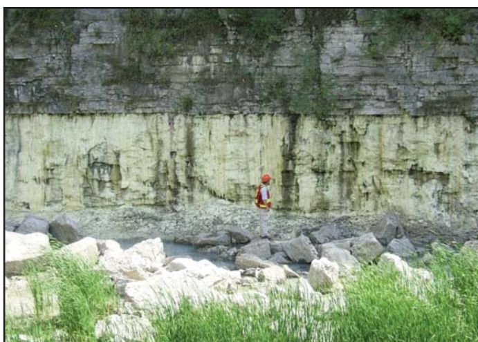
Figure 18. Water inflow along a horizontal bedding plane parting in limestone of the lower Dundee Formation, Port Dover Quarry. Yellow slime covering the quarry walls is a vigorous population of sulphur-oxidizing bacteria.
