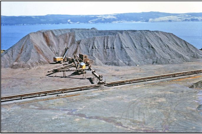
Figure 18. Conveyor and stockpile for ore storage adjacent to the Scotia pier. Source: Memorial University of Newfoundland–Digital Archives Initiative.
