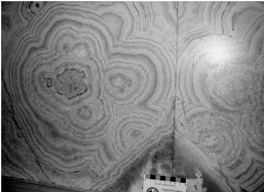
Figure 13 Egyptian travertine used in the side altar of the Blessed Virgin consisting of alternating concentric spherical bands of white and light brown calcite.
