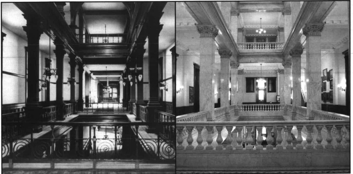
Figure 11 Wood floors, iron railings, and wood trim as seen in the left photo (City of Toronto Archives, Fonds 1244, Item 3003A) were replaced with concrete and marble floors of tesserae, and marble trim as seen in the photo on the right (Legislative Assembly of Ontario).
