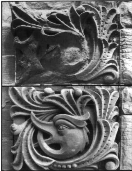
Figure 15 Before and after repair. Stonecarver Lawrence Voaides, created in Red St. Bees sandstone, the form of carving interpreted from that in the weathered Sackville sandstone
