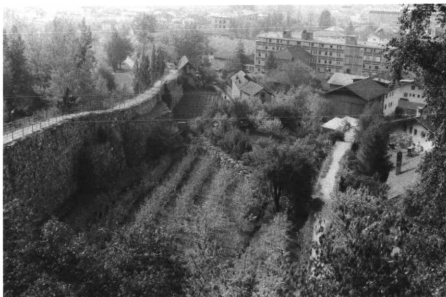
Figure 5 Two generations of protective debris-diversion dams at Schlanders, Italy. The older dam (on the right) was breached and practically buried during a debris flow catastrophe in 1731. A larger dam which eventually reached a length of 300 metres and a height of 10 metres (on the left) has served its purpose well since
