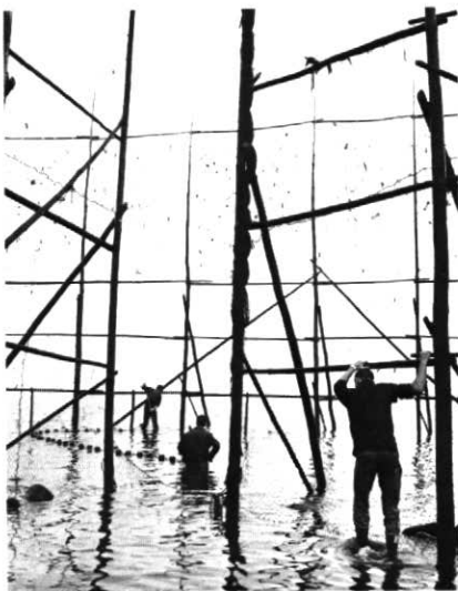
Figure 7 Fish weir at Halls Harbour in the Bay of Fundy. Note the sea weed caught near the top of the net at high tide. The maximum tidal range in the upper reaches of the Bay of Fundy is about 51 feet. (Photo from N.S. Communications and Information Centre.)
