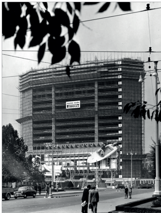
FIGS. 2-3. A STAGE IN THE CONSTRUCTION OF THE PIRELLI CENTRE: COMPLETION OF THE 17TH FLOOR. "PIRELLI FOR THE SEA" ADVERTISING INSTALLATION DESIGNED BY ROBERTO MENGHI AND ALBE STEINER, 1957 (LEFT) AND TYPICAL FLOOR PLANS (ABOVE), FROM A HIGHER FLOOR TO A LOWER FLOOR (TOP TO BOTTOM). | CAMERA-COLOR MILANO, COURTESY OF FONDAZIONE PIRELLI (LEFT), PLANS RETRACED BY KATIE FILEK (ABOVE).
