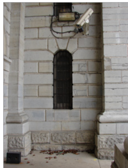
FIG. 15. COVERDALE, PROVINCIAL PENITENTIARY, NORTH GATE, 1843-1844; DETAIL OF ASHLAR AND BOTH VERMICULATED AND GROOVED RUSTICATION ON WALLS, PIERS, AND HALF PILASTERS OF PORTICO. | PHOTO: PAUL CHRISTIANSON, MARCH 2021.
