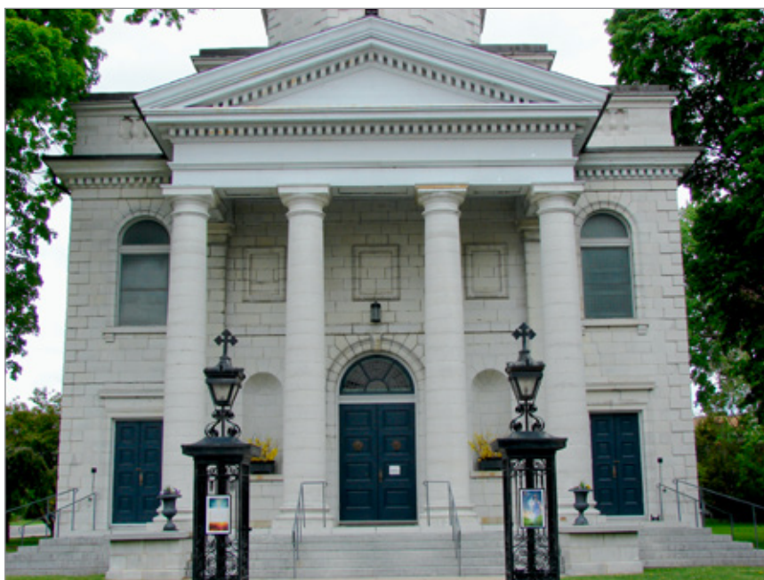
FIG. 37. ST. GEORGE'S CHURCH, RITUAL WEST FAÇADE, 1842; DETAIL OF STONEMWORK ON FAÇADE, PORTICO, AND STYLOBATE. | PHOTO: PAUL CHRISTIANSON, APRIL 2021.
