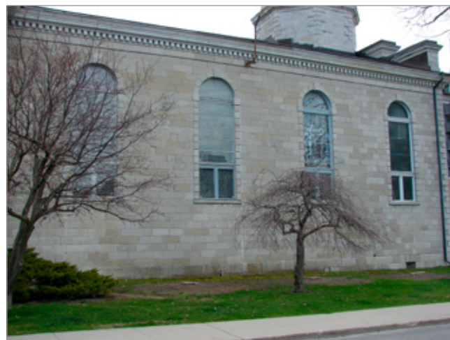
FIG. 4. ST. GEORGE'S CATHEDRAL, KINGSTON, ONTARIO, RITUAL SOUTH FAÇADE. DETAIL OF THREE BAYS FROM 1825-1826 AND ONE BAY FROM 1839-1841, ALL AS MODIFIED IN 1891. | PHOTO: PAUL CHRISTIANSON, APRIL 2020.
