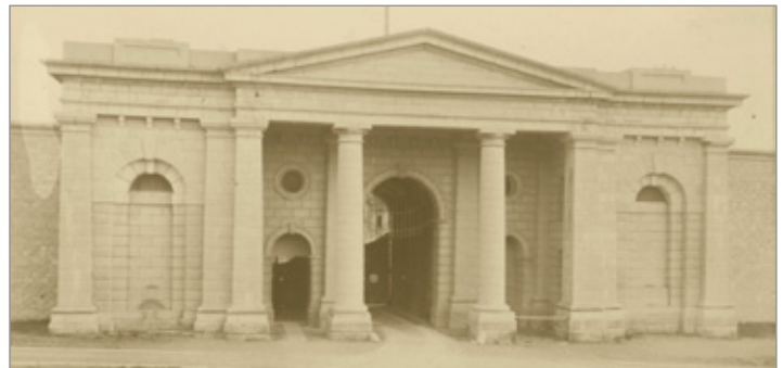
FIG. 6. WILLIAM COVERDALE, PROVINCIAL PENITENTIARY, DETAIL OF THE NORTH FAÇADE OF THE NORTH GATE, DESIGNED 1840 AND BUILT 1843-1844; PHOTO LATE 1800S. | SOURCE: QUA, KPC A-ARCH V23 PUB KINGSTON PEN #29. PHOTO: QUA.
