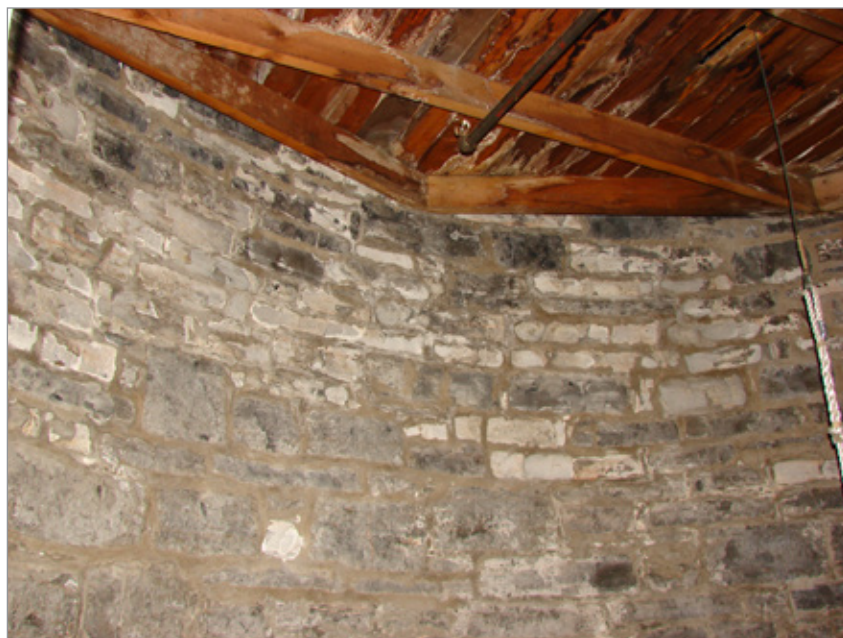
FIG. 18. ST. GEORGE'S CHURCH, 1839-1841; DETAIL OF THE INTERIOR OF THE TAPERED CIRCULAR WALL WHERE IT MEETS THE FLOOR OF THE BELFRY. | PHOTO: PAUL CHRISTIANSON, NOVEMBER 2020.
