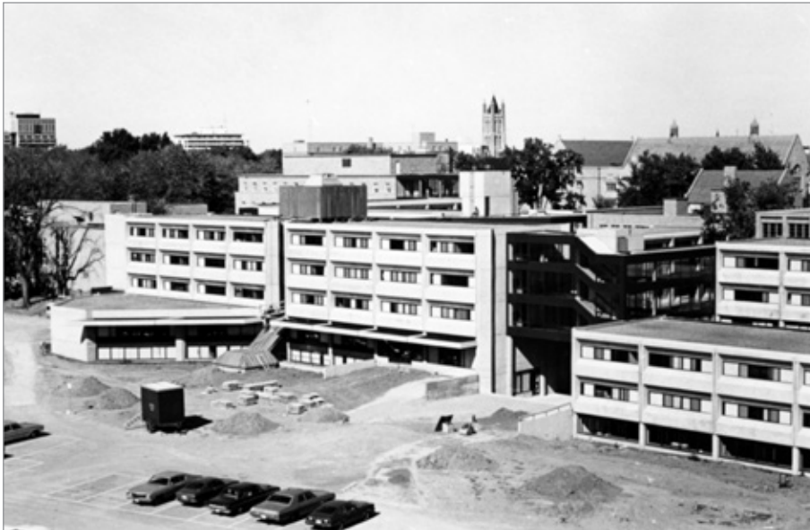
FIG. 7. VIEW OF ARTS AND SOCIAL SCIENCES COMPLEX (R.J. THOM ARCHITECTS, 1972-1974, TODAY MCINTOSH-CORRY HALL) LOOKING EAST, QUEEN'S UNIVERSITY, KINGSTON. | UNKNOWN PHOTOGRAPHER, C. 1974, QUEEN'S UNIVERSITY ARCHIVES, V28-B-MACKIN-4, QUEEN'S PICTURE COLLECTION, BUILDINGS, MACKINTOSH-CORRY HALL.
