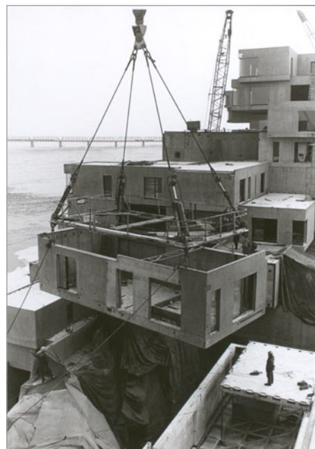
FIG. 19. GANTRY CRANE LIFTING MODULE INTO PLACE, 1966-1967. | SAFDIE ARCHITECTS. SOURCE: MOSHE SAFDIE FONDS, CANADIAN ARCHITECTURE COLLECTION, MCGILL UNIVERSITY LIBRARY, MONTREAL. COURTESY: SAFDIE ARCHITECTS.
