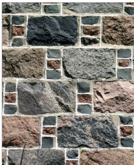
FIG. 16. CRELLIN'S ABERDEEN BOND STYLE MASONRY, WITH 3 SNECKS, MCCORQUODALE HOUSE, I 29 TH LINE, NO. 6565, NEAR HARRINGTON, OXFORD COUNTY. | KAREN E. ARMSTRONG.
