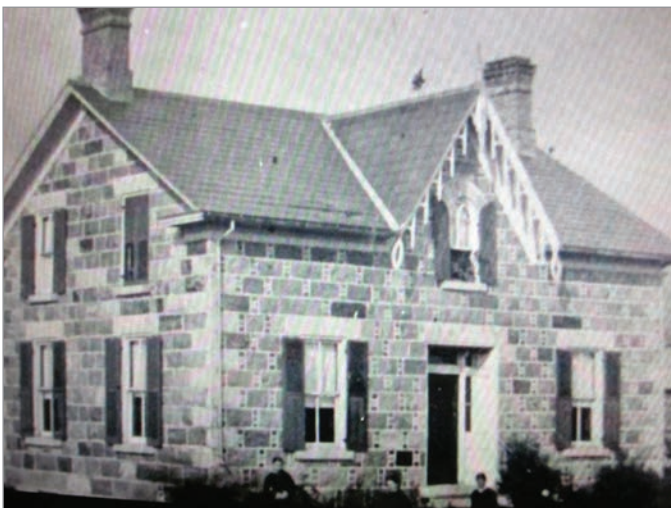
FIG. 11. MCCORQUODALE HOUSE, 29TH LINE, NO. 6565, NEAR HARRINGTON, OXFORD COUNTY. | UNDATED EARLY PHOTOGRAPH BY JOYCE GROVES.
