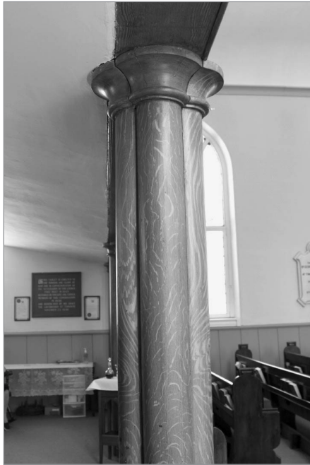
FIG. 31. GALLERY PIERS, HOLLAND LANDING. | ALANA DUGGAN.
