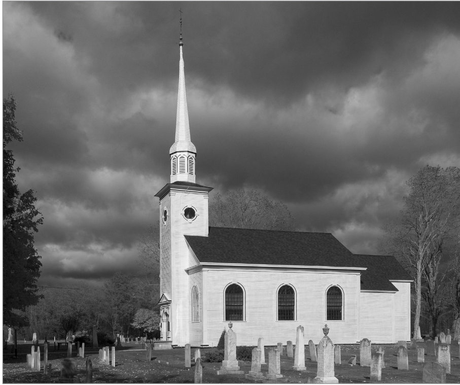
FIG. 4. ST. MARY'S CHURCH, AUBURN, NS, 1790. | PETER COFFMAN.
