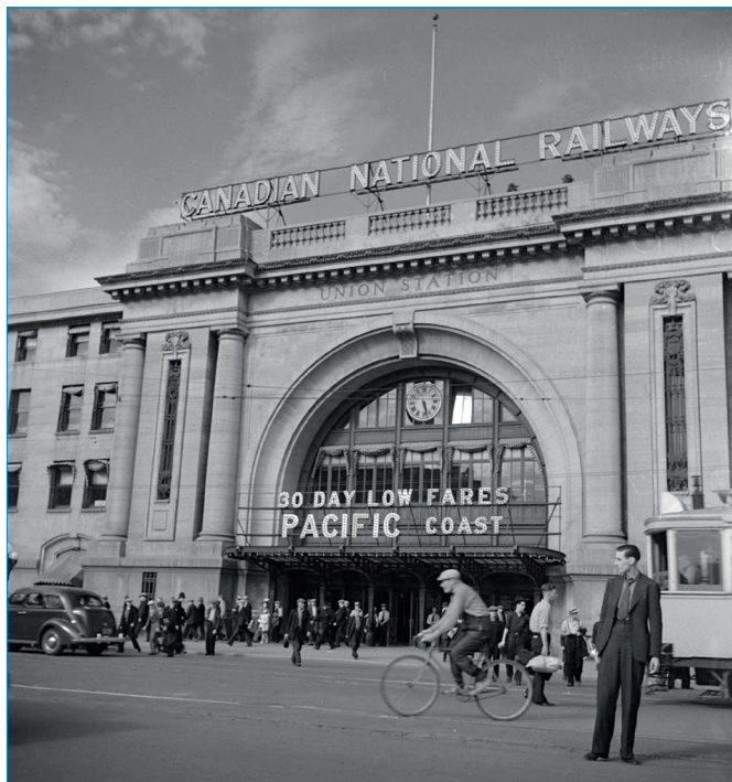
FIG. 13. CANADIAN NATIONAL RAILWAYS UNION STATION, WINNIPEG, WARREN & WETMORE, 1908-09, PHOTOGRAPHED C.1940-49. LIBRARY AND ARCHIVES CANADA / RONNY JAQUES FONDS / E010980620.
