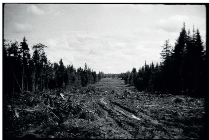
FIG. 6. CMHC ENGINEERING CREWS CLEARING ROAD CORRIDORS THROUGH THE THICK BUSH IN THE OROMOCTO TOWNSITE, 1954-1955. MAJOR ROADS WERE SEPARATED FROM ADJACENT HOUSING BY UNCLEARED BANDS OF FOREST. | CMHC PHOTO 1101-1124-013.
