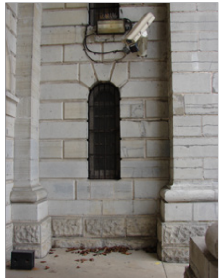
FIG. 15. COVERDALE, PROVINCIAL PENITENTIARY, NORTH GATE, 1843-1844; DETAIL OF ASHLAR AND BOTH VERMICULATED AND GROOVED RUSTICATION ON WALLS, PIERS, AND HALF PILASTERS OF PORTICO. | PHOTO: PAUL CHRISTIANSON, MARCH 2021.
