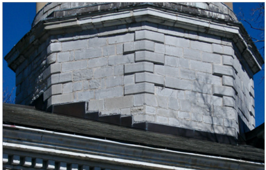
FIG. 16. ST. GEORGE'S ANGLICAN CHURCH, OCTAGONAL BASE OF TOWER, 1841-1842. | PHOTO: PAUL CHRISTIANSON, MAY 2022.
