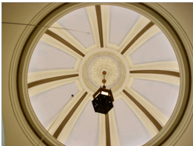
FIG. 31. ST. GEORGE'S ANGLICAN CHURCH, 1842; DETAIL OF MASONRY DOME IN THE CIRCULAR VESTIBULE. | PHOTO: PAUL CHRISTIANSON, NOVEMBER 2020.
