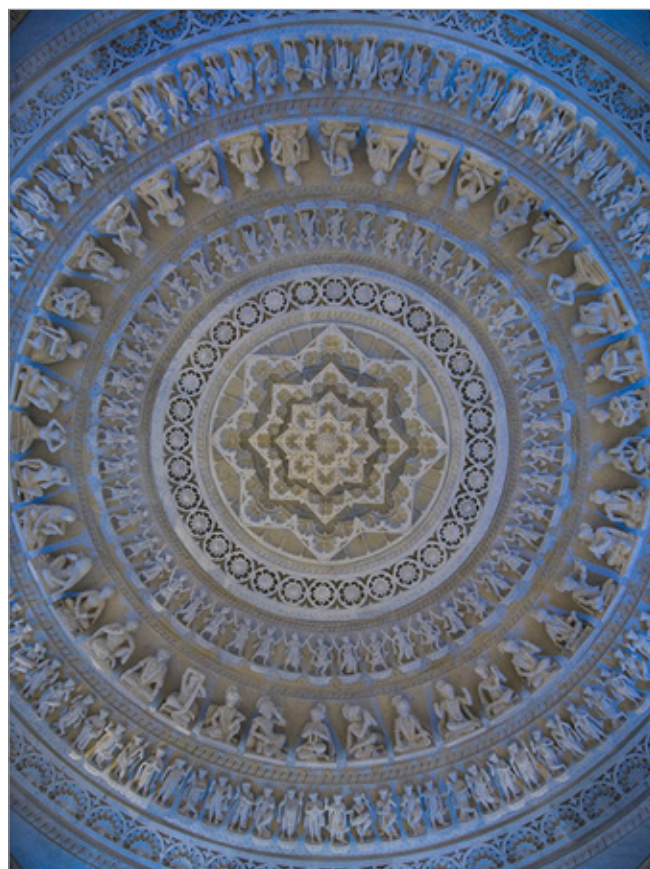
FIG. 13. CEILING OF CORBEL CONSTRUCTION USED TO TRANSITION FROM A SQUARE TO A CIRCLE. | BAPS TORONTO. COPYRIGHT HELD BY BAPS SWAMINARAYAN SANSTHA.
