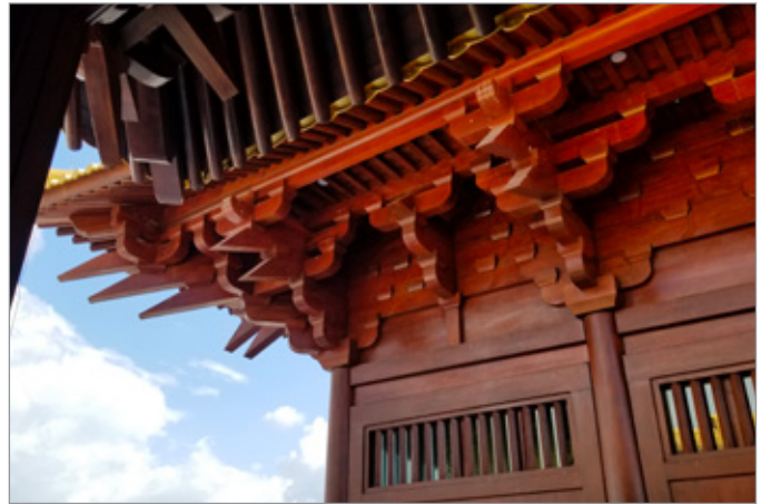
FIG. 21. AN EXTERIOR CLOSE-UP OF THE DOUGONG BRACKET SETS, MORTISE-AND-TENON CARPENTRY AND POST-AND-BEAM CONSTRUCTION USED IN THE MAIN DHARMA HALL AT THE WUTAI SHAN BUDDHIST GARDEN, 708 SKI HILL ROAD, BETHANY, ON. | EMILY J. GILBERT, AUGUST 2021.
