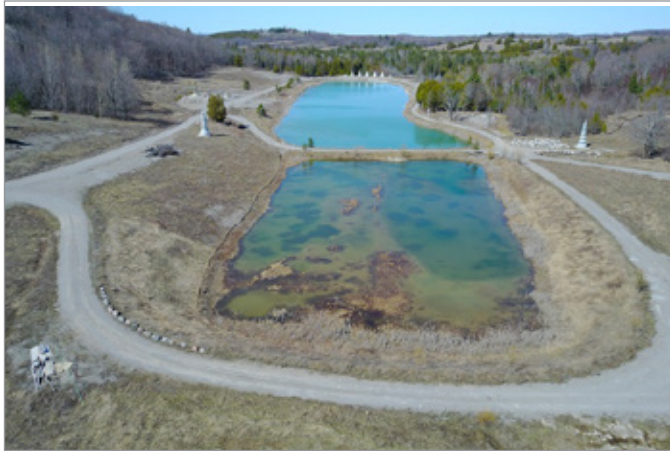
FIG. 28. CREATING WISDOM LAKE AT THE WUTAI SHAN BUDDHIST GARDEN, 708 SKI HILL ROAD, BETHANY, ON. | BUDDHIST ASSOCIATION OF CANADA'S CHAM SHAN TEMPLE: [HTTP://THEBUDDHISTGARDEN.COM/GALLERY%E7%9B%B8%E7%89%87%E9%9B%86/WISDOM-LAKE-%E9%9D%88%E6%B3%B9%E6%B9%96/], ACCESSED AUGUST 24, 2021.
