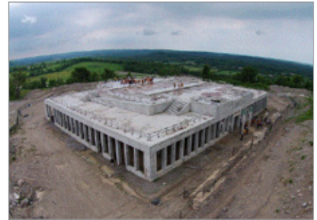
FIG. 19. THE STEEL AND REINFORCED CONCRETE LOWER LEVELS AND PLATFORM OF THE MAIN DARMA HALL AT THE WUTAI SHAN BUDDHIST GARDEN, 708 SKI HILL ROAD, BETHANY, ON. | BUDDHIST ASSOCIATION OF CANADA'S CHAM SHAN TEMPLE: [HTTP://THEBUDDHISTGARDEN.COM/GALLERY%E7%9B%B8%E7%89%87%E9%9B%86/MAIN-HALL-CONCRETE-FOUNDATION%E5%A4%A7%E6%AE%BF%E6%B0%B4%E6%B3%A5%E5%9F%BA%E7%A4%8E%E5%BB%BA%E8%A8%AD/], ACCESSED APRIL 5, 2021.
