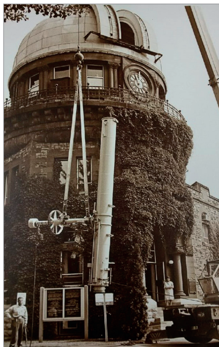
FIG. 10. FIFTEEN-INCH DOMINION TELESCOPE HOISTED FROM THE DOME OF THE DOMINION OBSERVATORY FOR TRANSFER TO CANADIAN SCIENCE AND TECHNOLOGY MUSEUM (CSTM), 1974. | DOMINION OBSERVATORY FONDS, BOX #2, CANADA MUSEUM OF SCIENCE AND TECHNOLOGY ARCHIVES, OTTAWA, CANADA.
