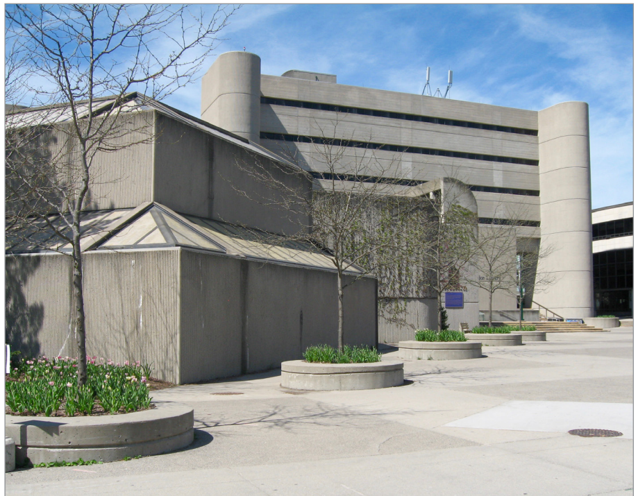
FIG. 9. THE SANDBLASTED, STRIATED CONCRETE WALLS OF THE D.B. WELDON LIBRARY (MURPHY, SCHULLER, GREEN, & MARTIN, AND JOHN ANDREWS ARCHITECTS), 2013, WESTERN UNIVERSITY, LONDON. | PHOTO: JAMES ASHBY.
