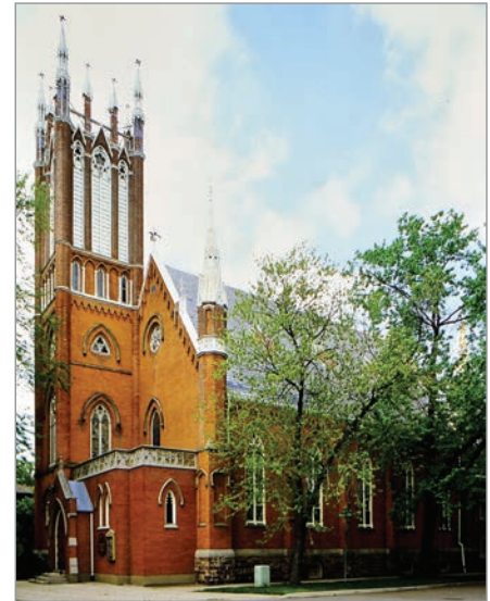
FIG. 37. ST. CATHARINES, WELLAND AVENUE METHODIST (UNITED) CHURCH, 1878, EXTERIOR. | MALCOLM THURLBY.
