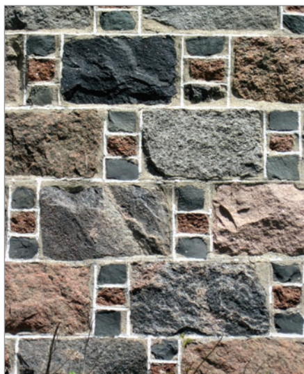
FIG. 16. CRELLIN'S ABERDEEN BOND STYLE MASONRY, WITH 3 SNECKS, MCCORQUODALE HOUSE, 1 29 TH LINE, NO. 6565, NEAR HARRINGTON, OXFORD COUNTY. | KAREN E. ARMSTRONG.
