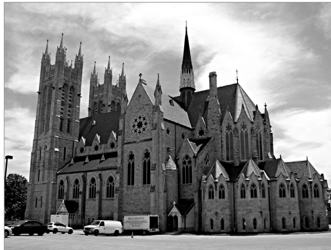
FIG. 3. VIEW OF SOUTH SIDE OF CHURCH OF OUR LADY OF THE IMMACULATE CONCEPTION IN GUELPH, ON (1876-1888). ARCHITECT: JOSEPH CONNOLLY. | KRISTIE DUBÉ.
