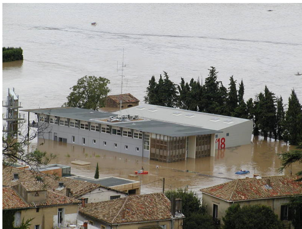
Figure 4. La caserne inondée / Firehouse flooded
