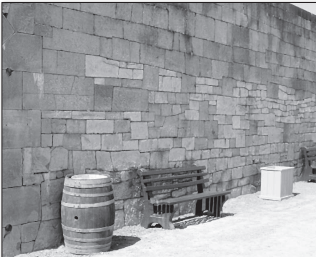
Figure 8: River wall at Fort Niagara showing the work of two contractors. Photo by the author.
