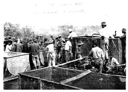
Figure 2. Cementing a Well in Miri.
