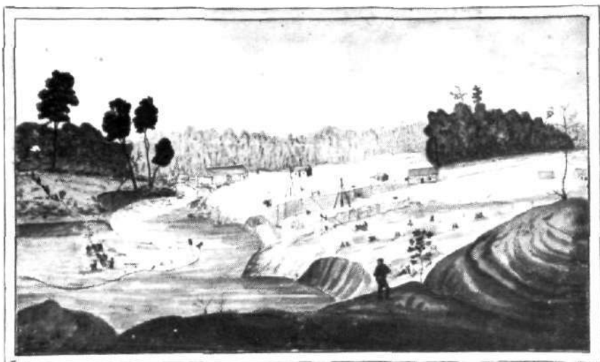
Brewers Lower Mill; excavations of canal and construction of locks in progress; note the barrow run on the left side of the picture; Burrowes Sketch, Archives of Ontario
