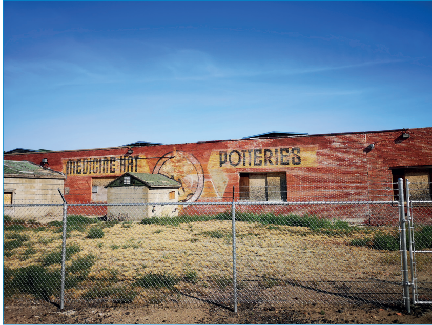
FIG. 5. FENCED-OFF WALL OF AN ABANDONED CLAY FACTORY IN MEDICINE HAT, SEPTEMBER 2022. BANAFSHEH MOHAMMADI.
