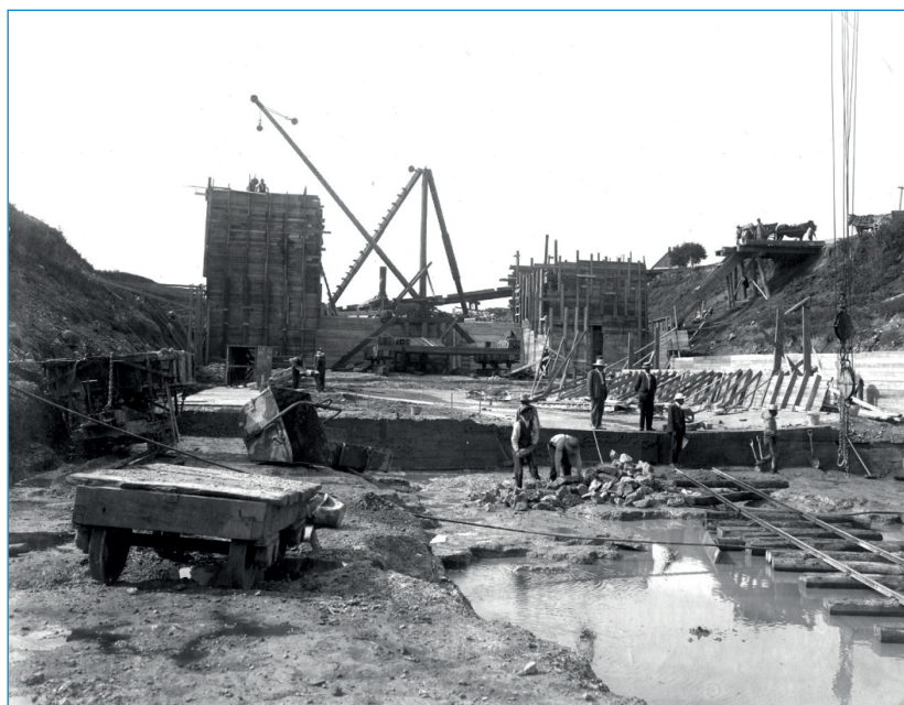
FIG. 6. PREPARATION WORK FOR ST. ANDREW'S LOCK AND DAM, LOCKPORT, MANITOBA. H. E. VAUTELET (DESIGN ENGINEER), 1900–1910, PHOTOGRAPHED IN 1908. ARCHIVES OF MANITOBA PHOTOGRAPH COLLECTION. 1984-129. LOCKPORT 28, CONSTRUCTION, 1908, P1188, N17222.
