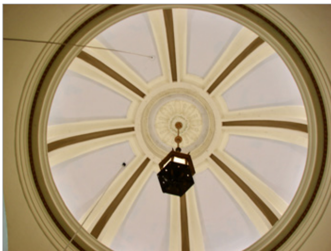
FIG. 31. ST. GEORGE'S ANGLICAN CHURCH, 1842; DETAIL OF MASONRY DOME IN THE CIRCULAR VESTIBULE. | PHOTO: PAUL CHRISTIANSON, NOVEMBER 2020.
