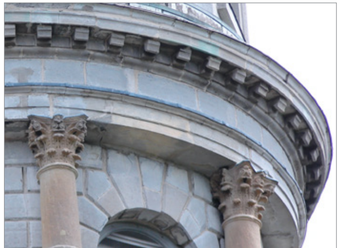
FIG. 49. ST. GEORGE'S CHURCH, BELFRY, 1842; DETAIL OF CORINTHIAN CAPITALS AND ENTABLATURE. | PHOTO: PAUL CHRISTIANSON, JULY 2022.
