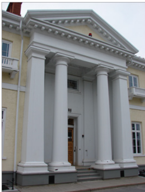
FIG. 22. GEORGE BROWNE, ROCKWOOD VILLA, HATTERS BAY (NOW KINGSTON), 1841; DETAIL OF TUSCAN PORTICO. | PHOTO: PAUL CHRISTIANSON, MAY 2020.
