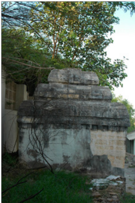
FIG. 18. THE HORIZONTAL LAYERING AND PYRAMIDICAL FORM OF THE PHAṂSANĀ STYLE OF ŚIKHARA AT THE SEVENTH-CENTURY TEMPLE NUMBER TWO, MIYĀNĪ, GUJARAT, INDIA. | LIBBIE MILLS, DECEMBER 2010.
