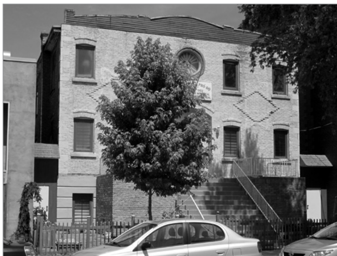
FIG. 6. THE EXTERIOR TODAY OF POALE ZEDEK ON URBAIN STREET, MONTRÉAL, AN EXCEPTIONAL SYNAGOGUE THAT WAS PHYSICALLY DESIGNED AND BUILT BY THE CONGREGANTS ON AND OFF BETWEEN 1910 AND 1922. | BARRY L. STIEFEL, MAY 2010.
