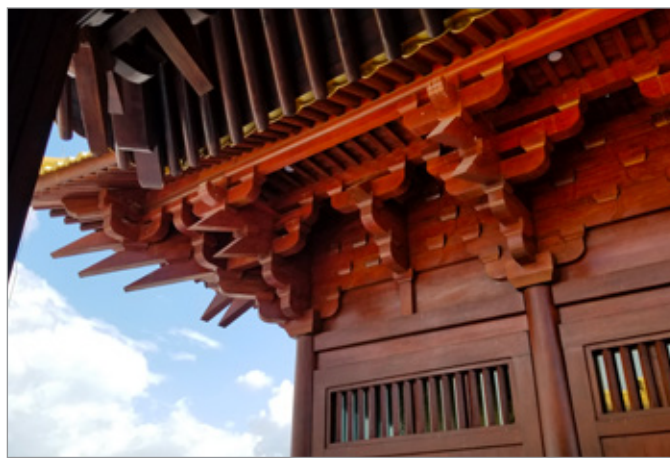
FIG. 21. AN EXTERIOR CLOSE-UP OF THE DOUGONG BRACKET SETS, MORTISE-AND-TENON CARPENTRY AND POST-AND-BEAM CONSTRUCTION USED IN THE MAIN DHARMA HALL AT THE WUTAI SHAN BUDDHIST GARDEN, 708 SKI HILL ROAD, BETHANY, ON. | EMILY J. GILBERT, AUGUST 2021.
