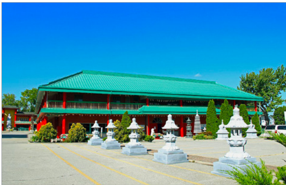
FIG. 14. ADJACENT TO THE BUDDHIST ASSOCIATION OF CANADA'S TEN THOUSAND BUDDHAS SARIRA [RELICS] STUPA, THE CONTRASTING HALL OF FIVE CONTEMPLATIONS TEMPLE, 4303 RIVER ROAD, NIAGARA FALLS, ON. | ROY W., PUBLIC DOMAIN, TRIPADVISOR: [HTTPS://WWW.TRIPADVISOR.CA/ATTRACTION_REVIEW-G154998-D3547891-REVIEWS-CHAM_SHAN_TEMPLE-NIAGARA_FALLS_ONTARIO.HTML#MEDIA-ATFJ3547891/223255794/P?ALBUMID=-160&TYPE=0&CATEGORY=-160], ACCESSED AUGUST 24, 2021.
