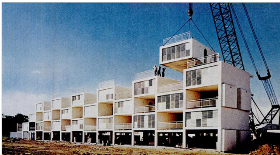
FIG. 21. VIVIENDA 70, SAN JUAN, PUERTO RICO, AUGUST KOMENDANT, CONSULTANT FOR SHELLEY SYSTEM, C. 1970. | UNKNOWN PHOTOGRAPHER. SOURCE: UNKNOWN.
