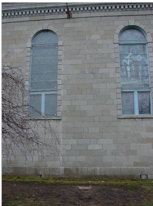
FIG. 6. TWO MODIFIED NAVE WINDOWS AND STONE WALL FROM THE SECOND ST. GEORGE'S ANGLICAN CHURCH. | PAUL CHRISTIANSON, JANUARY 2020.
