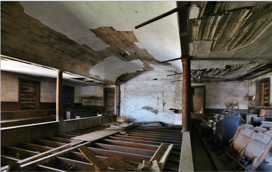
FIG. 5. BEAVERDAMS METHODIST CHAPEL, 1834, INTERIOR FROM SW GALLERY. | MALCOLM THURLBY.
