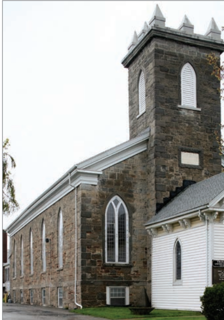
FIG. 15. THOROLD, TRINITY WESLEYAN METHODIST (UNITED) CHURCH, 1845, EXTERIOR FROM NW (SE). | MALCOLM THURLBY.
