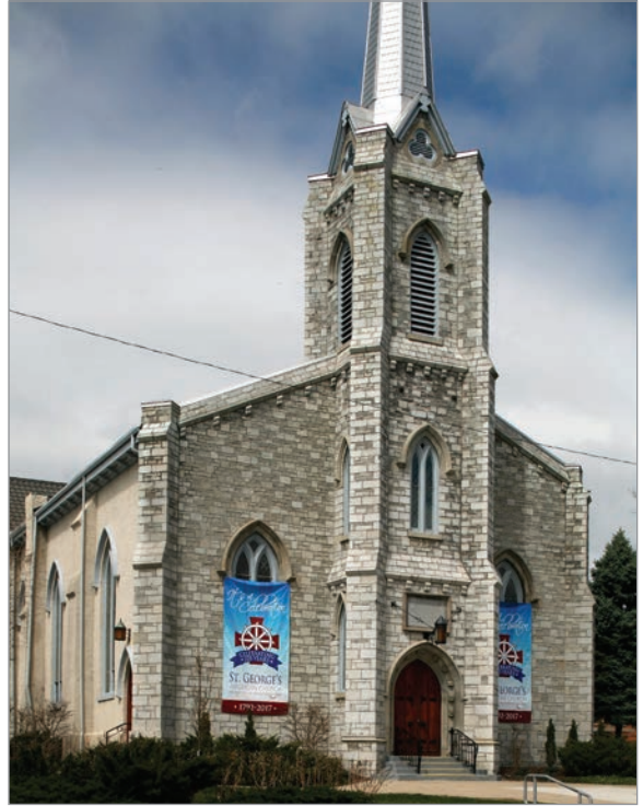
FIG. 11. ST. CATHARINES, ST. GEORGE'S ANGLICAN CHURCH, 1844, EXTERIOR. | MALCOLM THURLBY.
