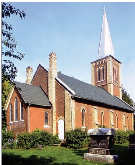
FIG. 22. MCNAB, CHRIST CHURCH ANGLICAN, EXTERIOR NE. | MALCOLM THURLBY.
